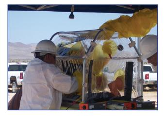
Glovebags are soft-sided enclosures that form a small work area to confine the spread of contamination. The use of glovebags can help you attain your ALARA goals by reducing your radiological waste and area of contamination.
